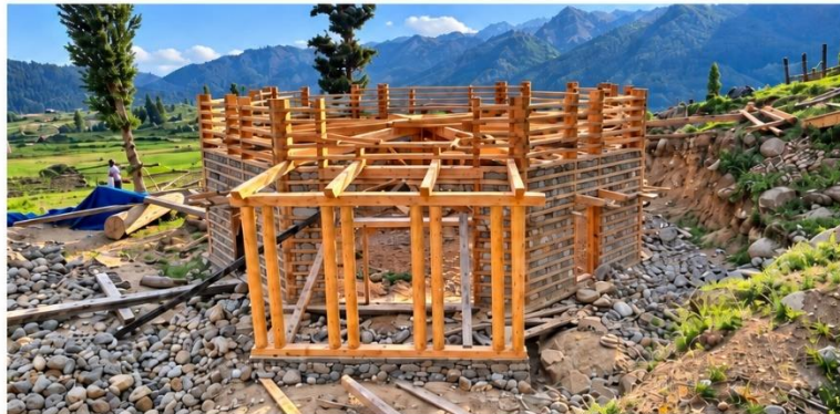
Figure 2.1. Timber laced stone masonry during construction (Location: Diamir; Photos Credit: Engr. Noshad Khan).
