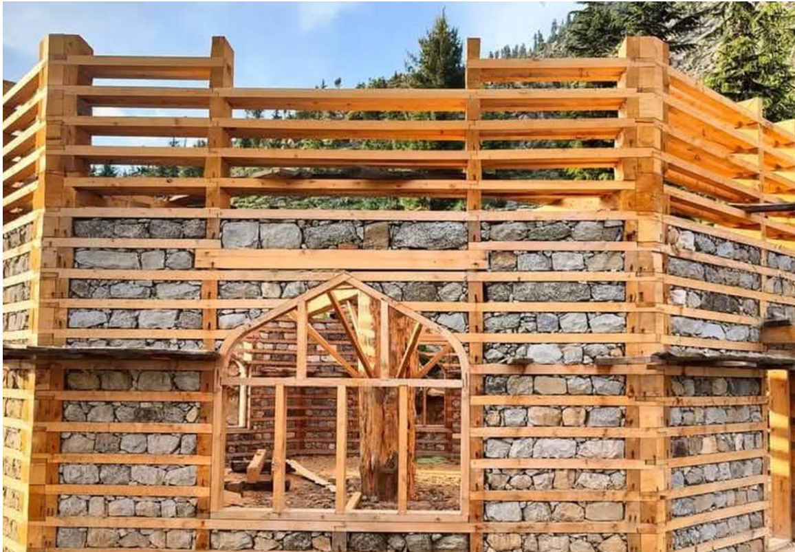
Figure 6.7. Continuous timber bands at wall corners (Location: Diamir; Photo Credit: Engr. Noshad Khan).
