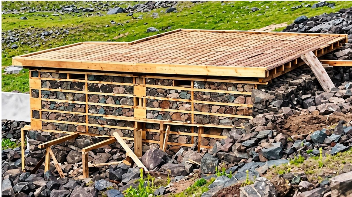
Figure 8.1. Completed hybrid stone timber houses (Location: Kohistan; Photo Credit: Engr. Ayub Khan).
