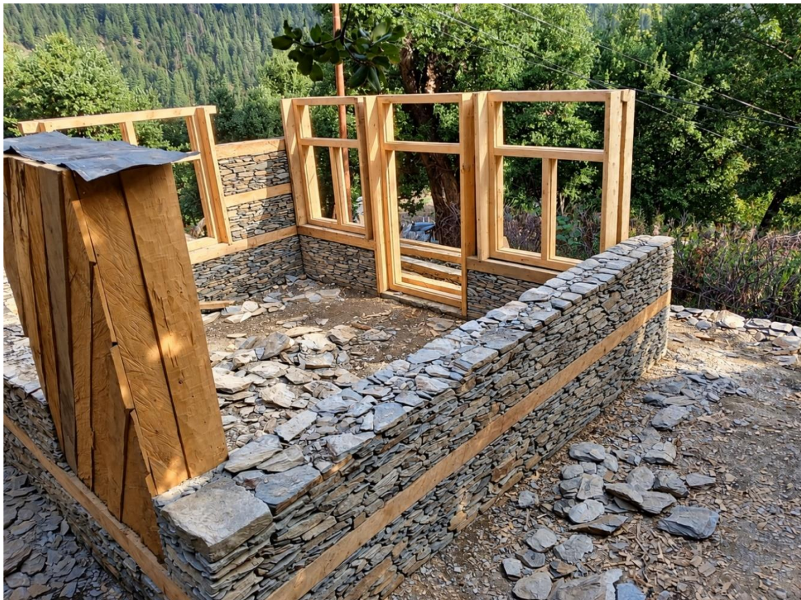
Figure 6.8. Timber framed openings in stone masonry (Location: Chitral; Photo Credit: Engr. Faheem Ul Jalal).
