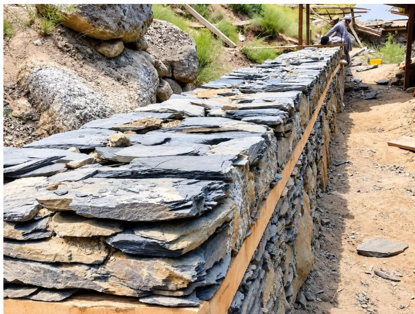
Figure 6.5. Bonded flat stone masonry with a timber band (Location: Chitral; Photo Credit: Engr. Faheem Ul Jalal).
