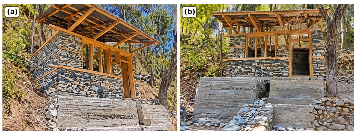
Figure 7.6. Hybrid stone timber buildings with reinforced concrete plinths (Location: Chitral; Photos Credit: Engr. Faheem Ul Jalal).
