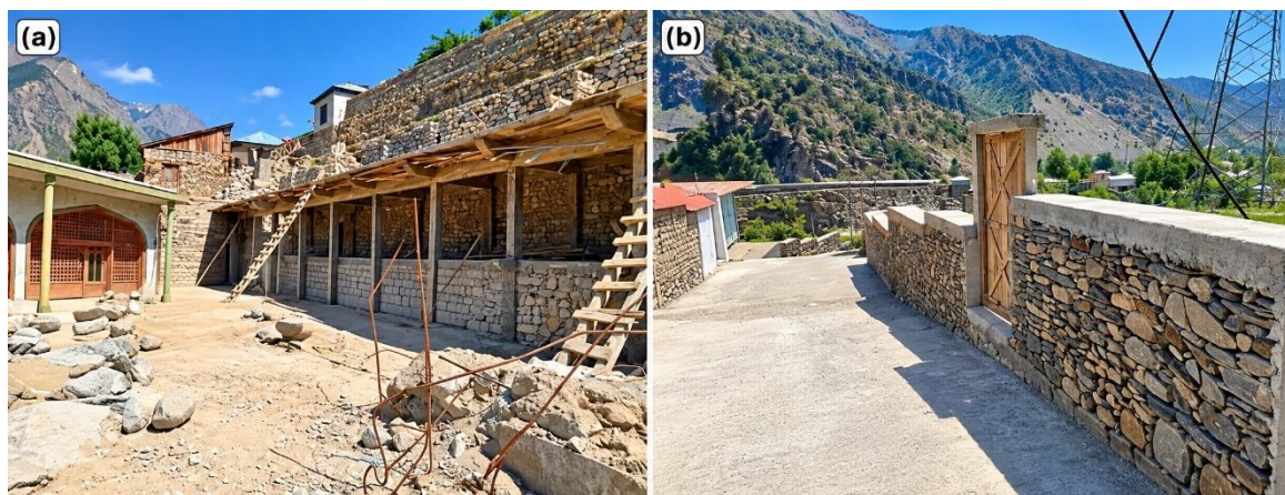
Figure 4.3. Field examples of variable stone masonry workmanship (Location: Diamir (a) & Chitral (b); Photos Credit: Engr. Noshad Khan & Engr. Faheem Ul Jalal).
