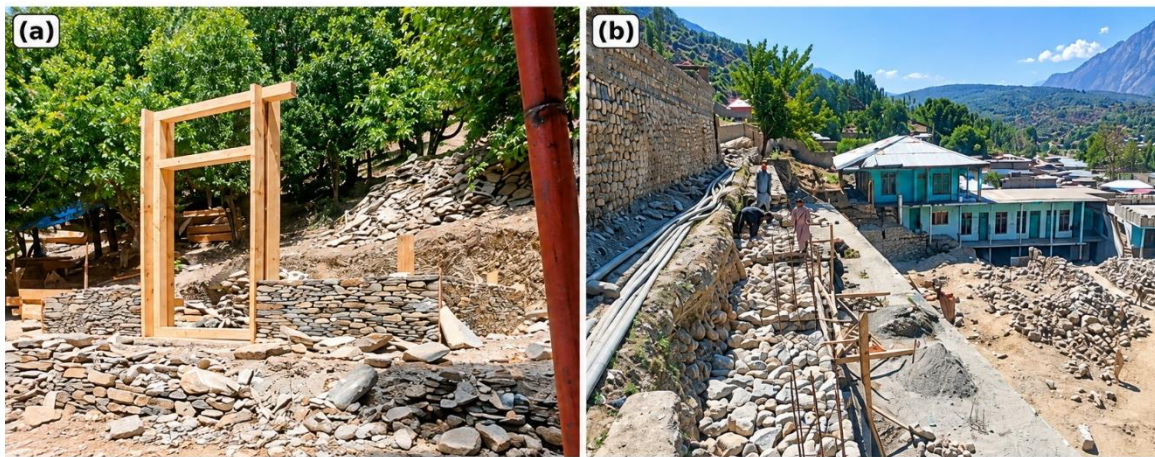
Figure 6.3. Foundation and plinth construction on sloping ground (Location: Chitral & Diamir; Photos Credit: Engr. Faheem Ul Jalal & Engr. Noshad Khan).
