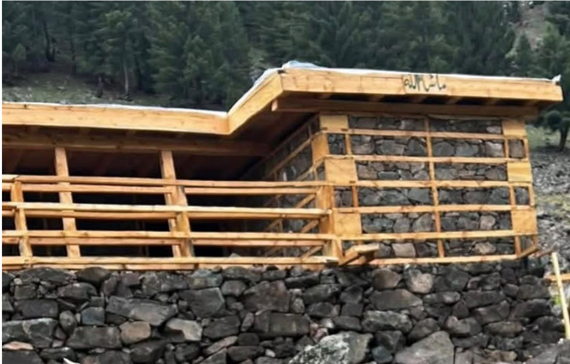
Figure 2.3. Completed timber laced stone house (Location: Kohistan; Photo Credit: Engr. Ayub Khan).
