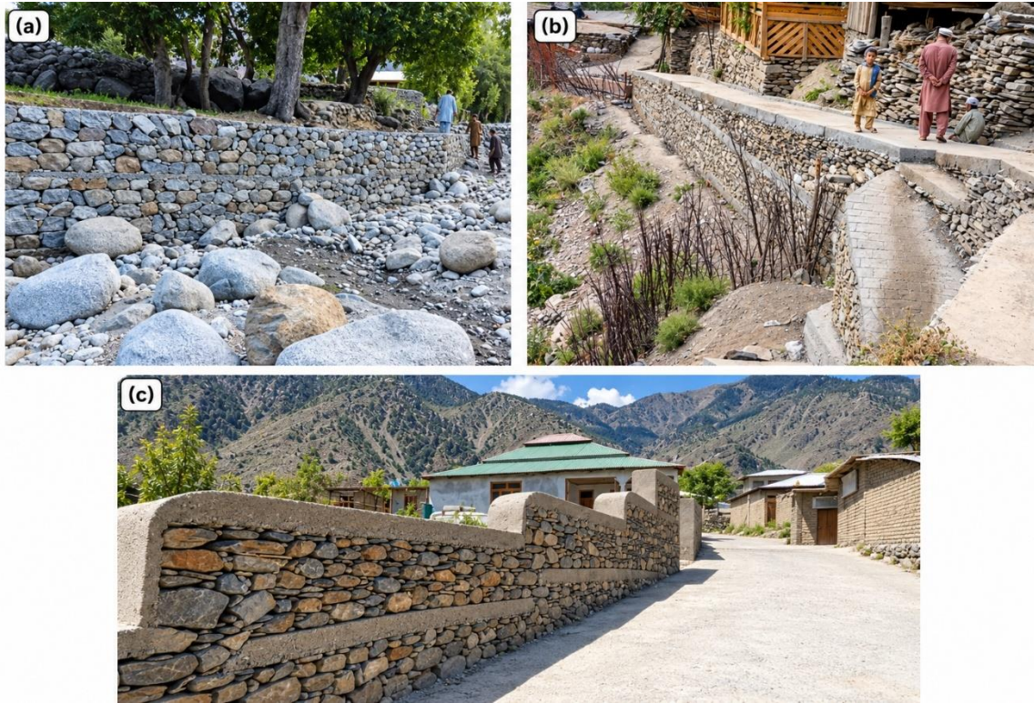
Figure 5.5. Field examples of slope support and retaining wall conditions (Location: Diamir & Chitral; Photos Credit: Engr. Noshad Khan & Engr. Faheem Ul Jalal).
