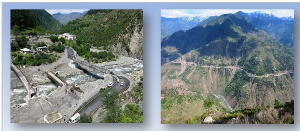
Figure 10: Examples of 2. Order road type: Kaghan valley near Paras (left) and close to Bala Kot (right);
